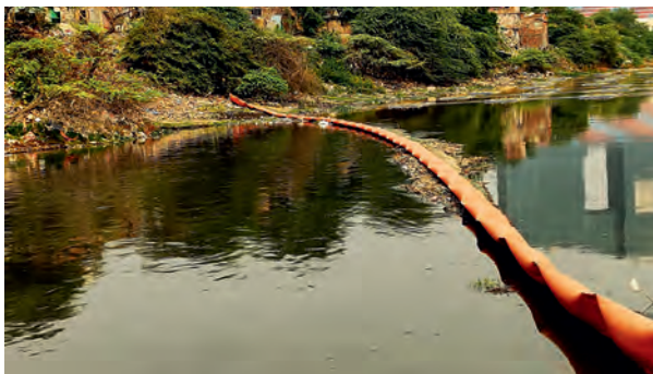
➤ Installed trash barriers, curtailing floating waste from falling into the Yamuna River, sustaining the local ecology
